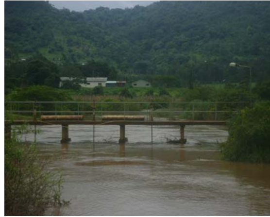
Photo 2: Intake Weir Site during high flow at end of June
